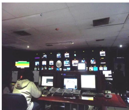
‘Control Room’ of Metro TV Jakarta
