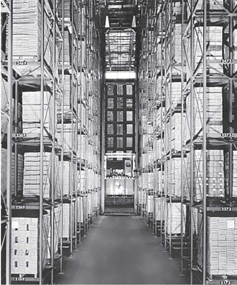
Figure 1.1 The first automated high-bay warehouse installed by Demag at the Bertelsmann publishing house in Wetter, Germany in 1962
