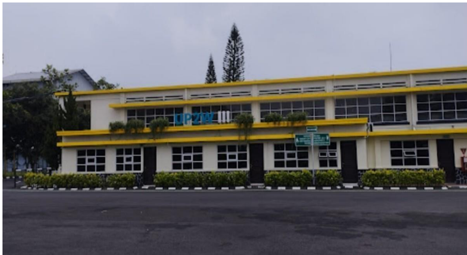
Gambar 1.0.1 Kantor PLN PUSHARLIS UP2W3
