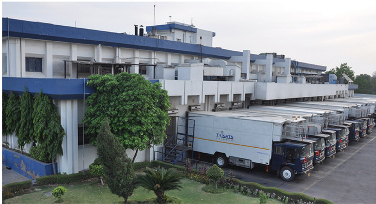
Figure 9.34 Building of TAJ-SATS Flight Kitchen, Madras
