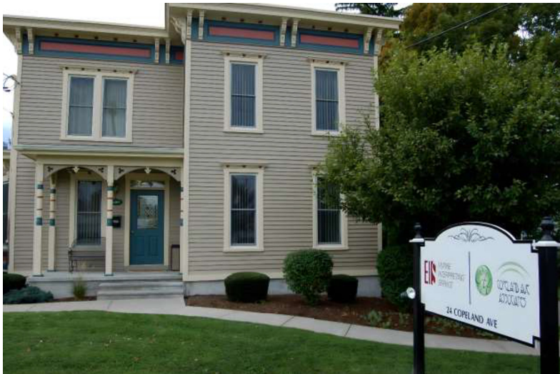
Figure 53.1 Building in Homer, NY, purchased to house my business
