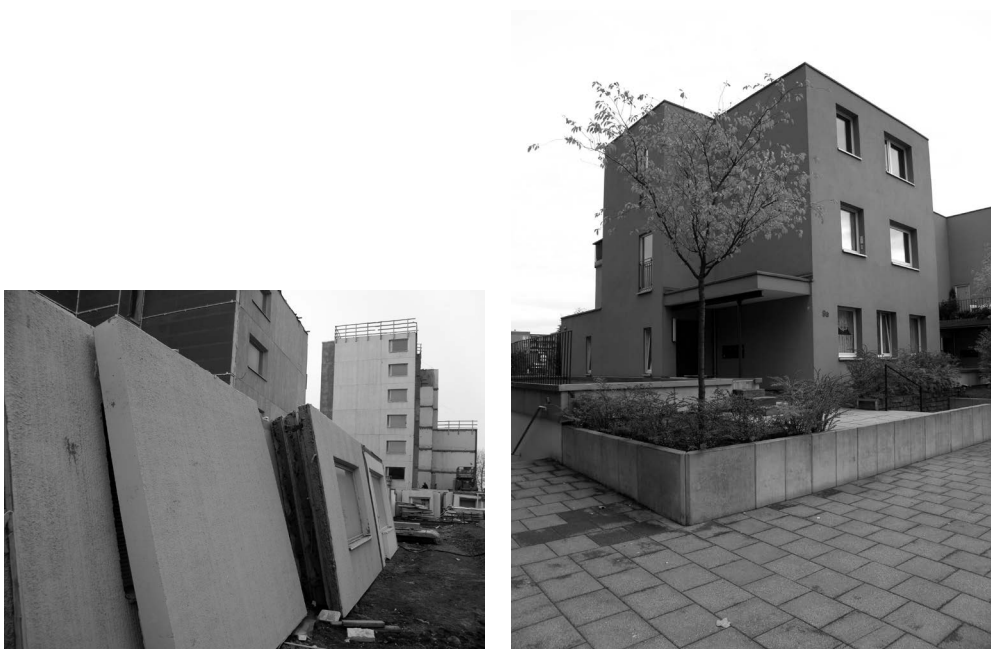
Figure 3.1 Concrete elements deconstructed from the buildings behind them (left). Location: Finland. A new building made from deconstructed elements (right). Location: Germany. Photos: SH.
