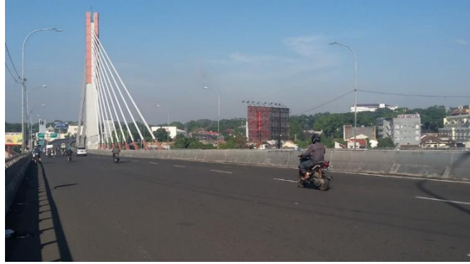
Figure 4. 7 Jalan Layang Pasopati (Source: Private Document, 2024)
