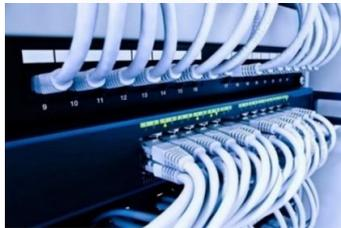
Gambar 2.5 Kabel LAN UTP (Unshielded Twisted Pair) [8]
