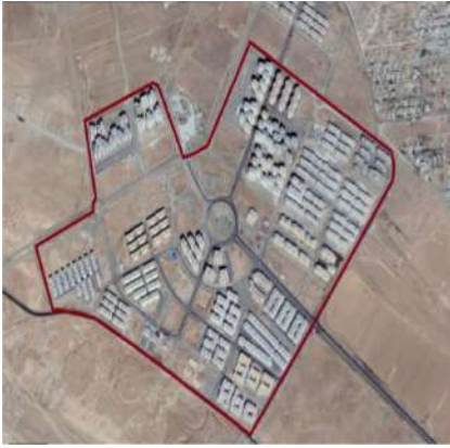
Fig. 9. Site (c) (Google earth, 2020)
