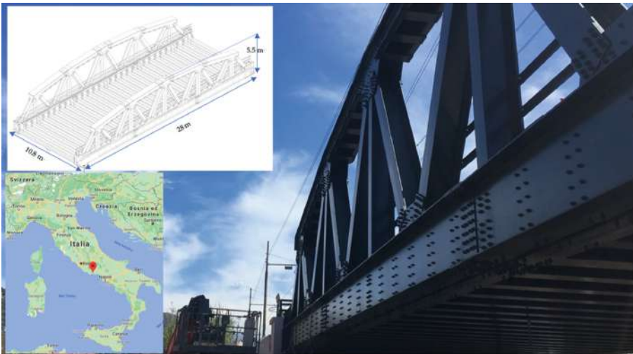
Fig. 1. The Portella bridge
