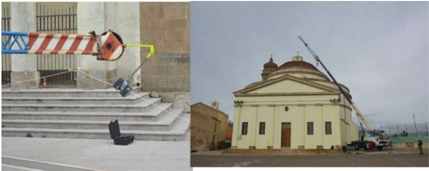
Fig. 3. TLS survey of the roof
