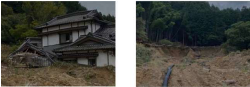
Fig. 4. Landslide field in Soeda-Cho, Japan
