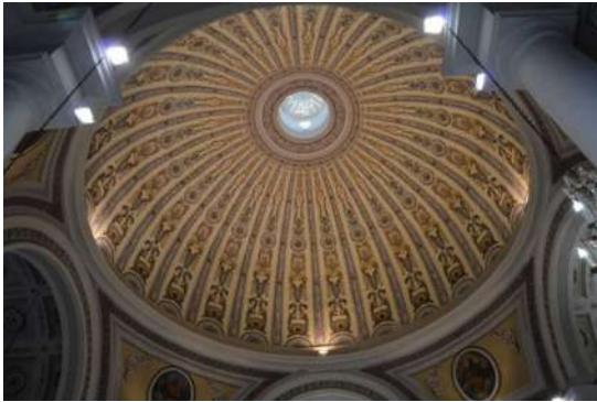
Fig. 8. Internal view of the dome.
