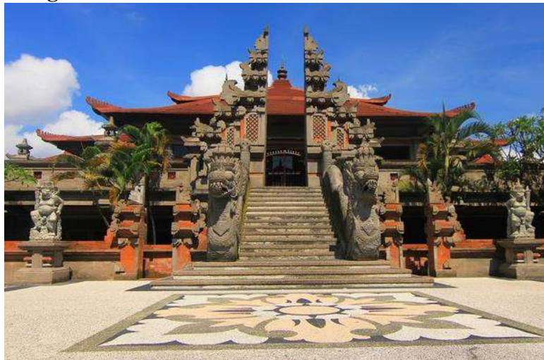
Gambar. 35 – Gedung Ksiranawa (Sumber: indonesiakaya.com, 2021)
