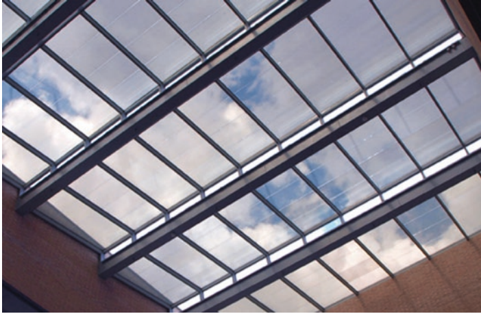
Fig. 31.3 Innovative transparent PV panels [4]
