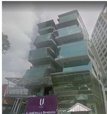
Gambar 13. Fasad U Janevalla sumber: Google Street View
