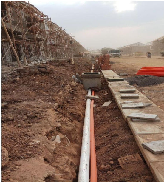
Gambar 1.1 Proyek Ducting fo-sr
