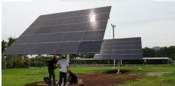
Gambar 2. 1 Single axis solar tracker
