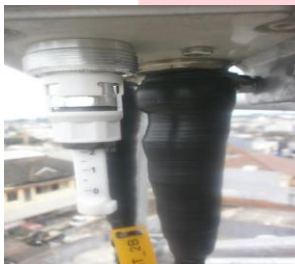
Gambar 2.6 Electrical downtilt
