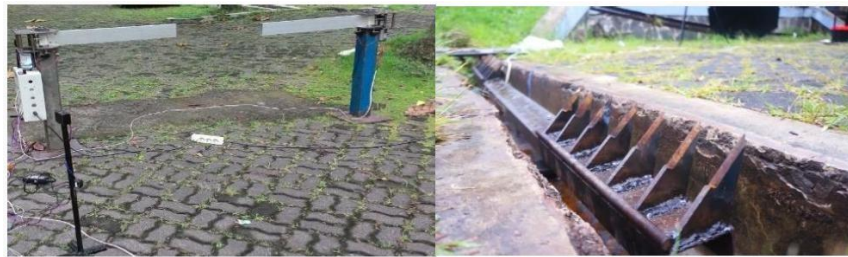
Gambar 4. 1 Implementasi main gate dan security gate
