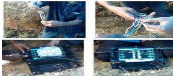
Gambar 4.3 Proses Penyambungan di Fussion Splicer
