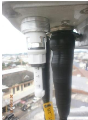
Gambar 2.8 Electrical downtilt
